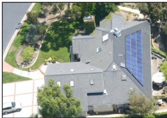
PV Solar Panel Roof
