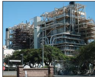
AES Power Plant
